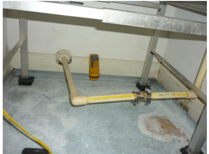
Area view of the photo to the left
